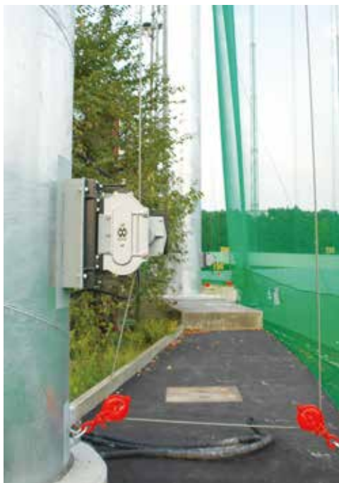
▲ Raising and Lowering the Nets at Golf Driving Range
